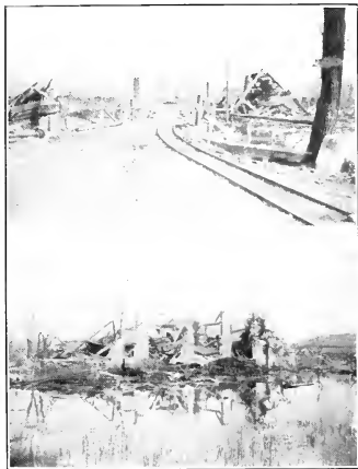
Bridge over Vesle River. Mill at Villette.
